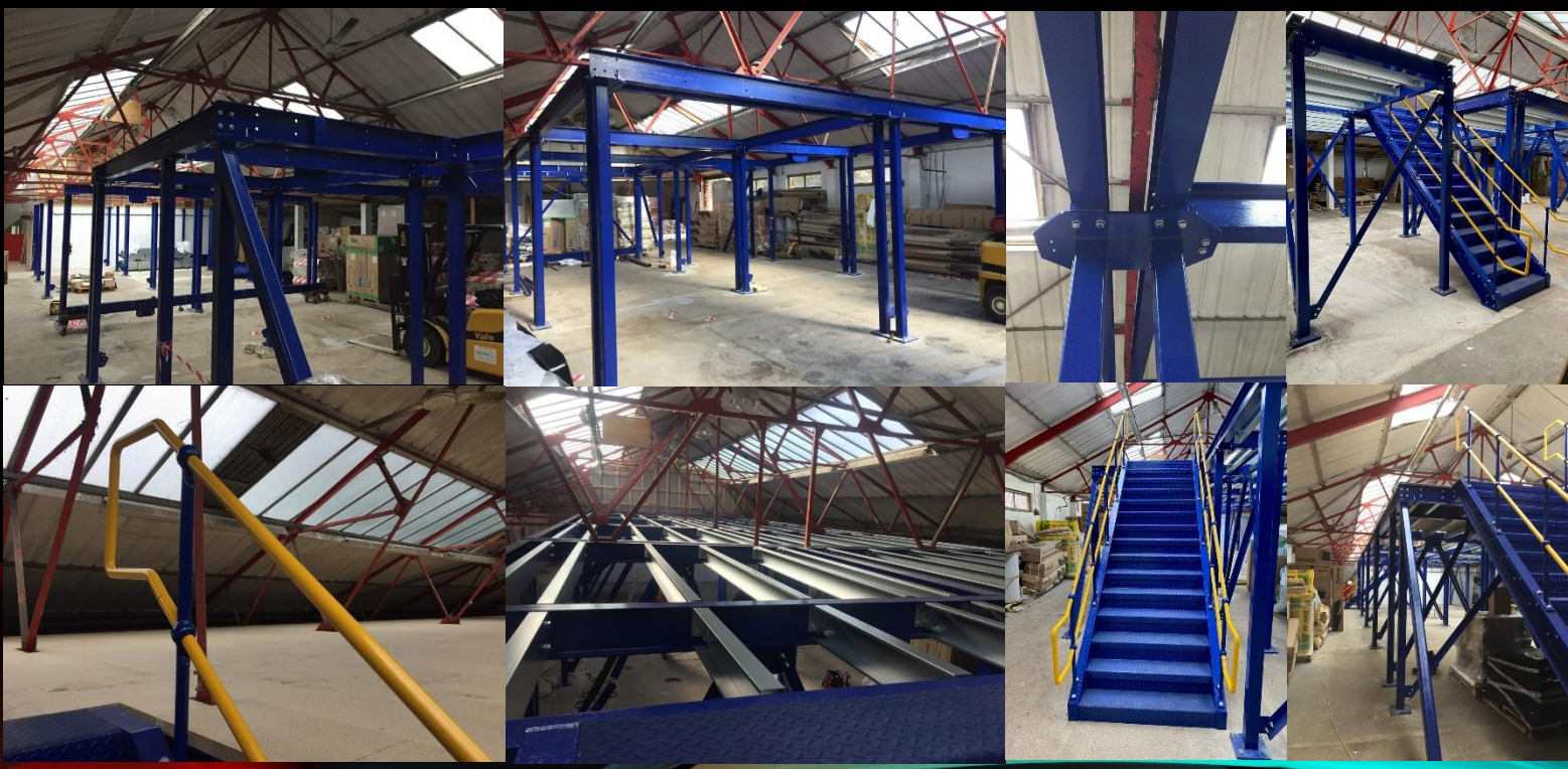
Images of the Installed Mezzanine Floor.
